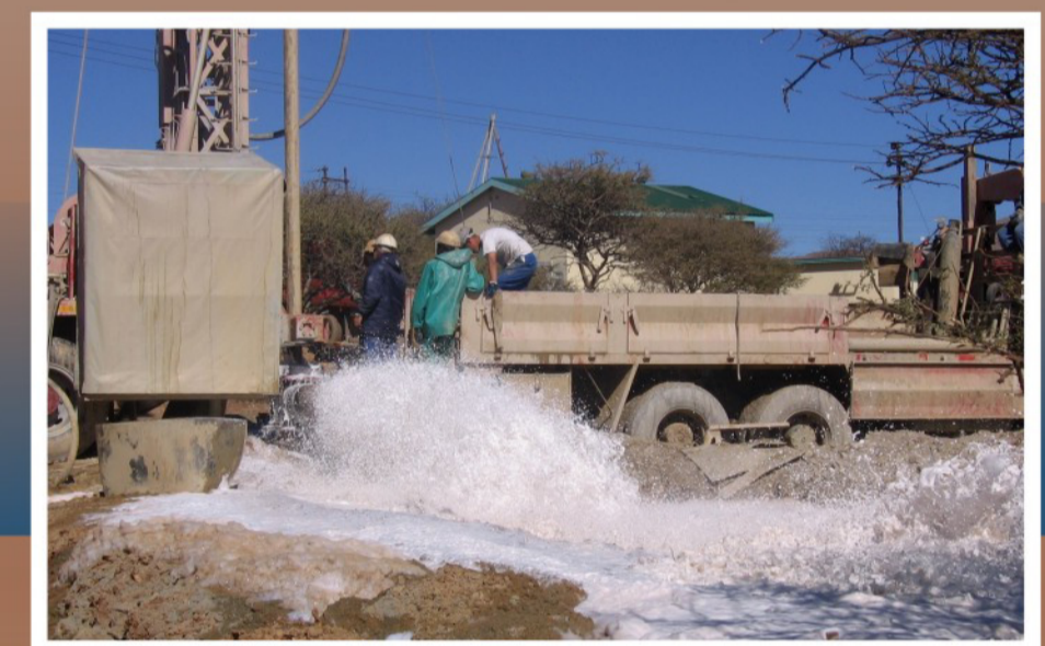
Drilling deep (500m) abstraction boreholes, Windhoek, Namibia
