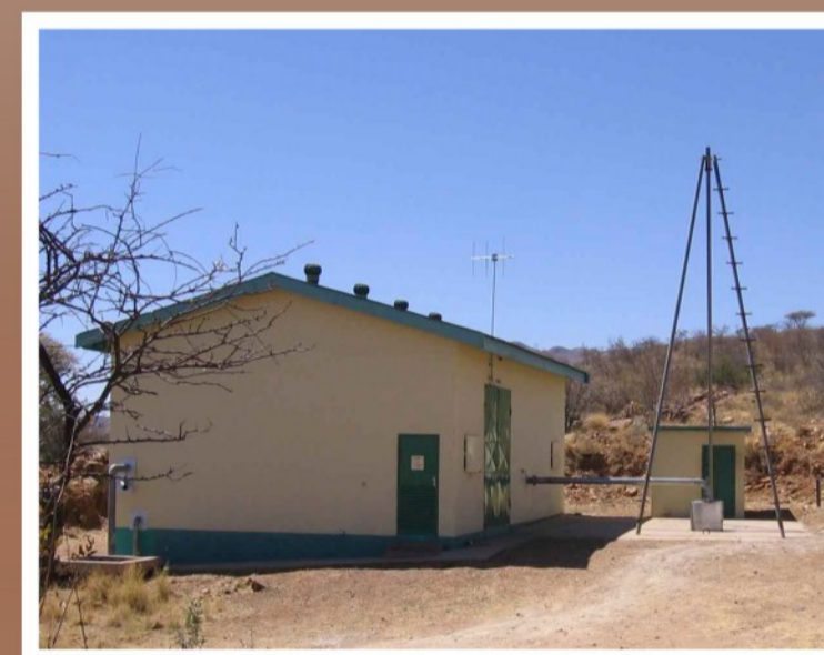
Injection borehole, Windhoek, Namibia
